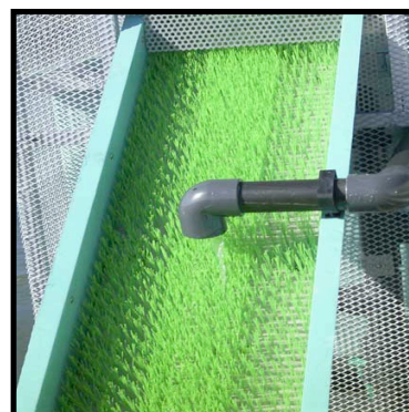
Rampe de reptation (MRM)
